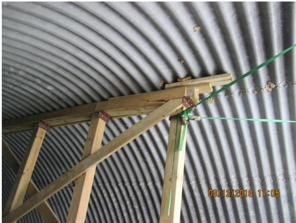
Timber bracing displaying cracking/splitting
