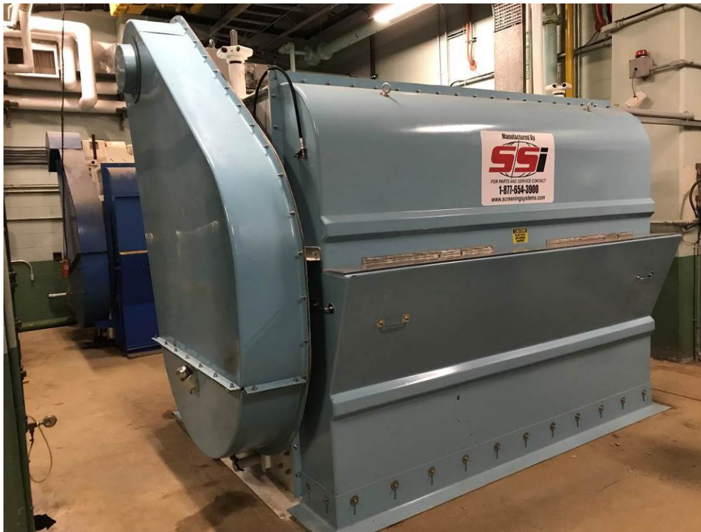
Figure 6: New travelling screen #2 in the low lift pump station.
