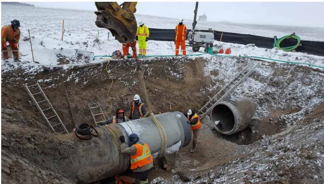
Figure 8c: Installation of the first repair piece.
