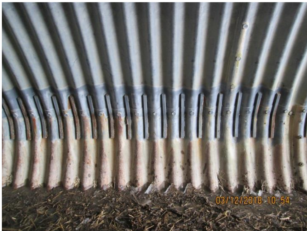
Crack reinforcement along south side of structure
