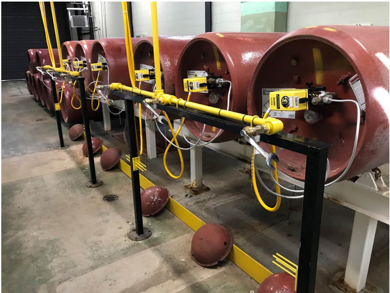
Figure 5: The chlorine gas tonners, fitted with emergency electric actuated operators.
