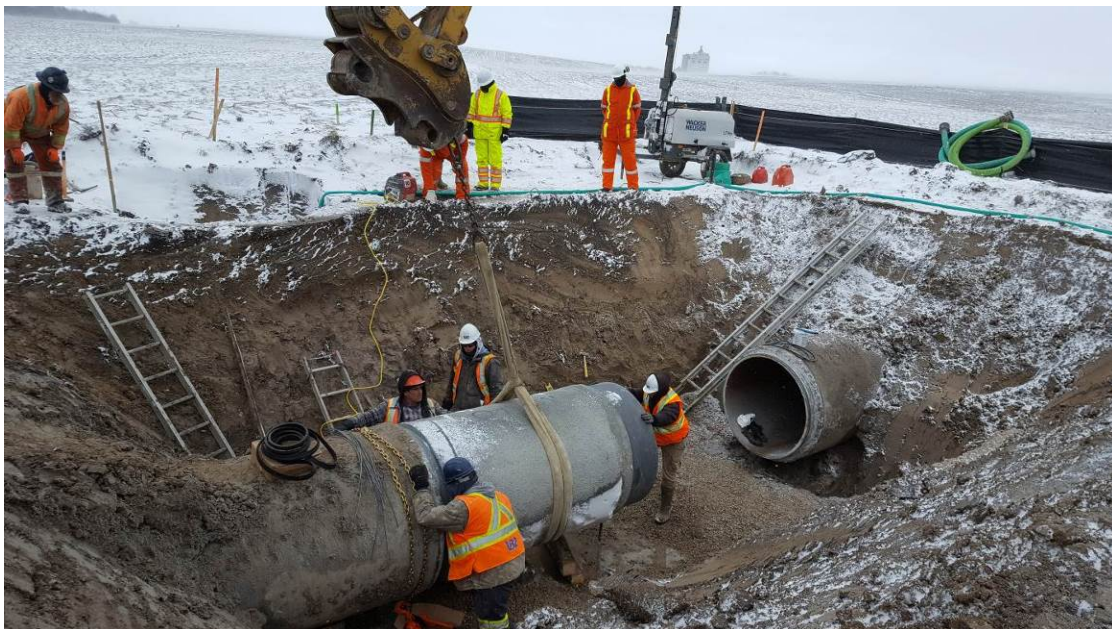
Figure 8c: Installation of the first repair piece.
