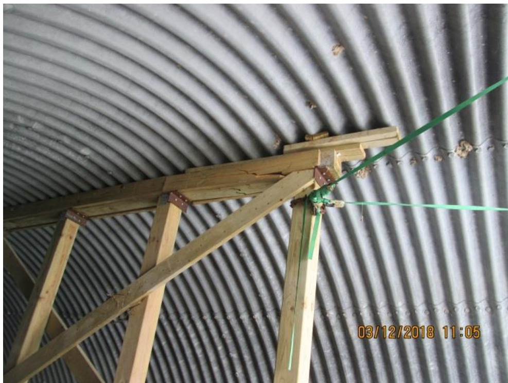
Timber bracing displaying cracking/splitting
