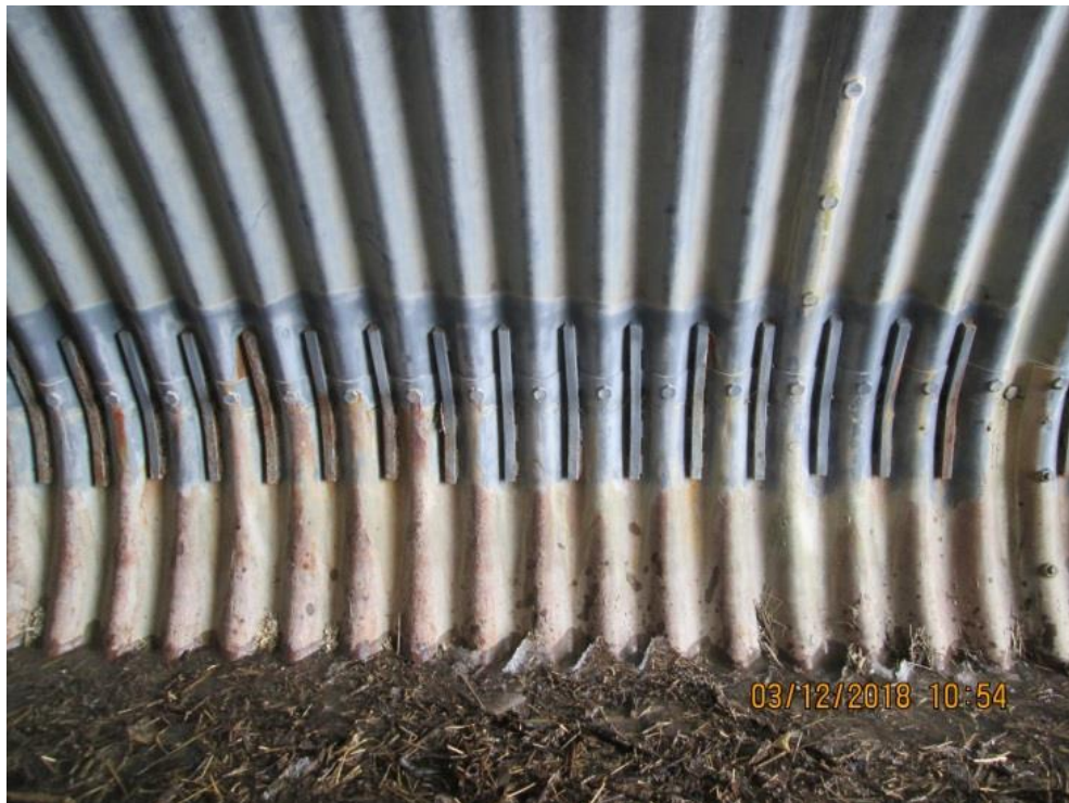
Crack reinforcement along south side of structure
