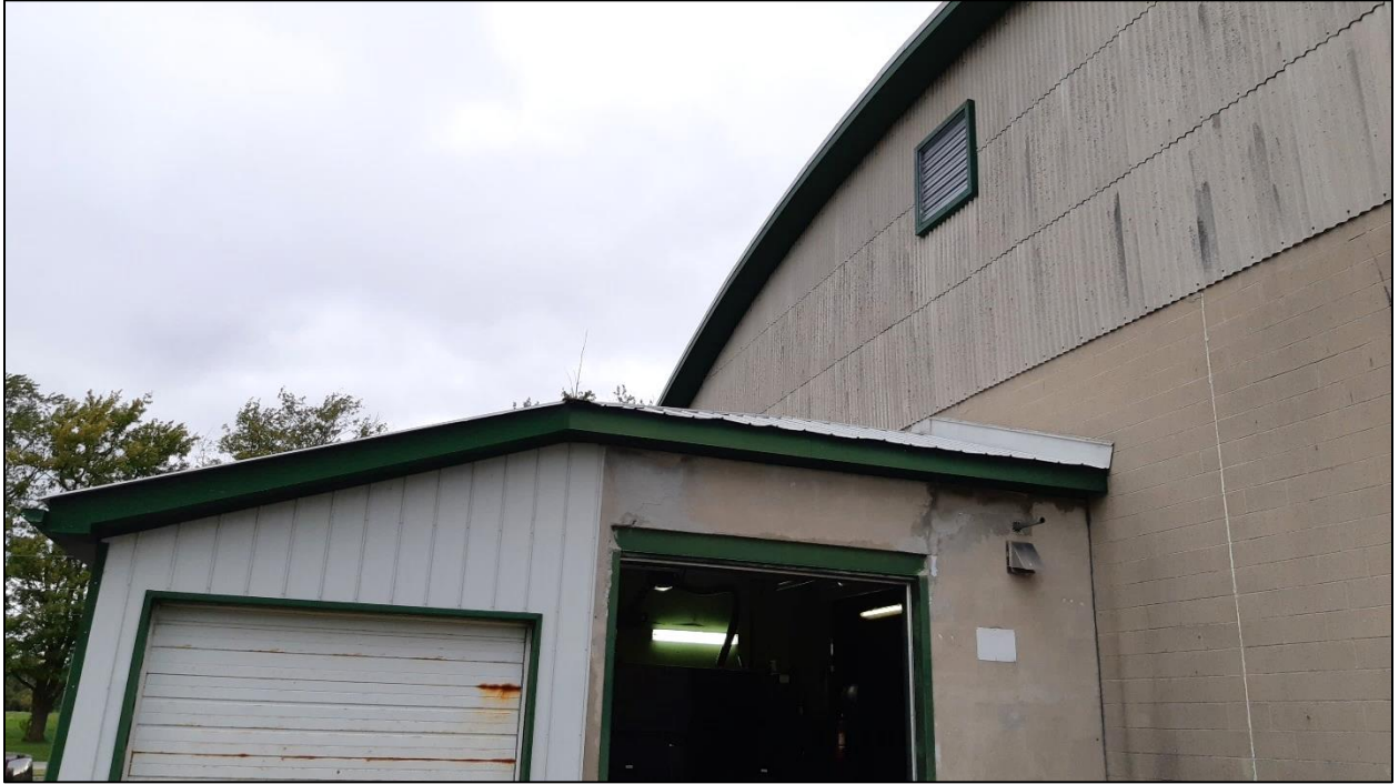
Height Differential between Shed/Olympia Room and Arena
