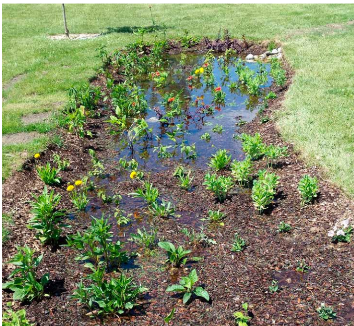
Rain water soaks into the ground in one of the rain gardens.
