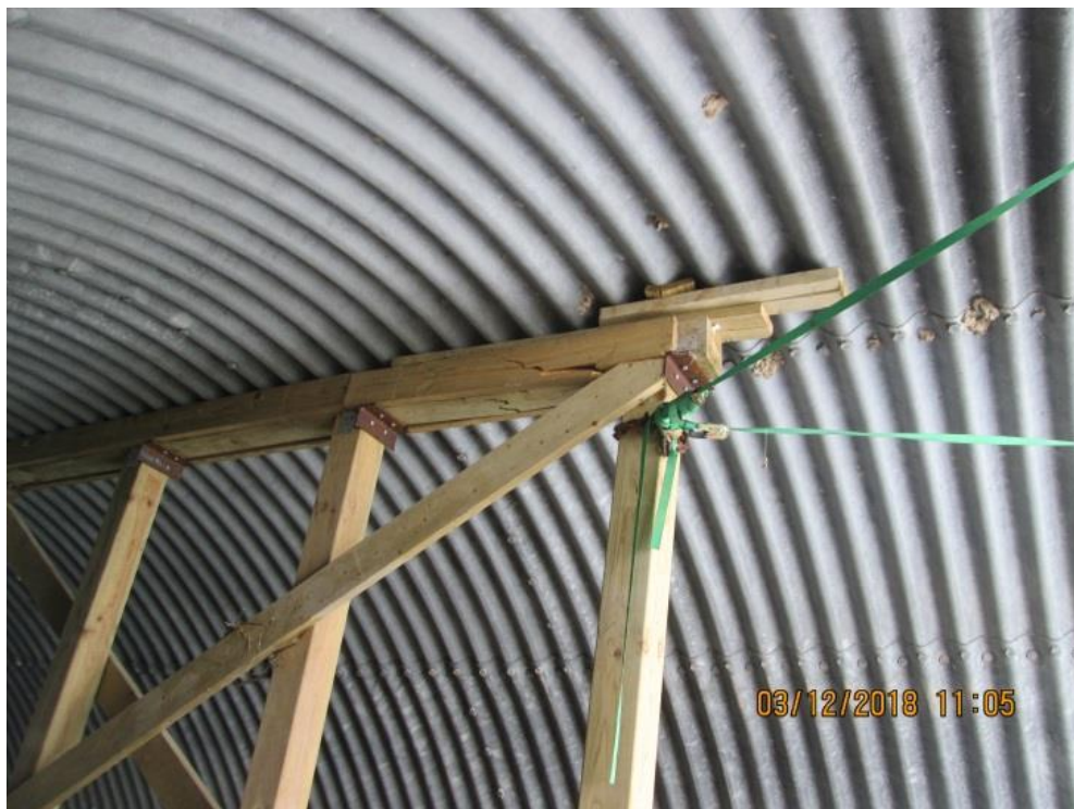
Timber bracing displaying cracking/splitting
