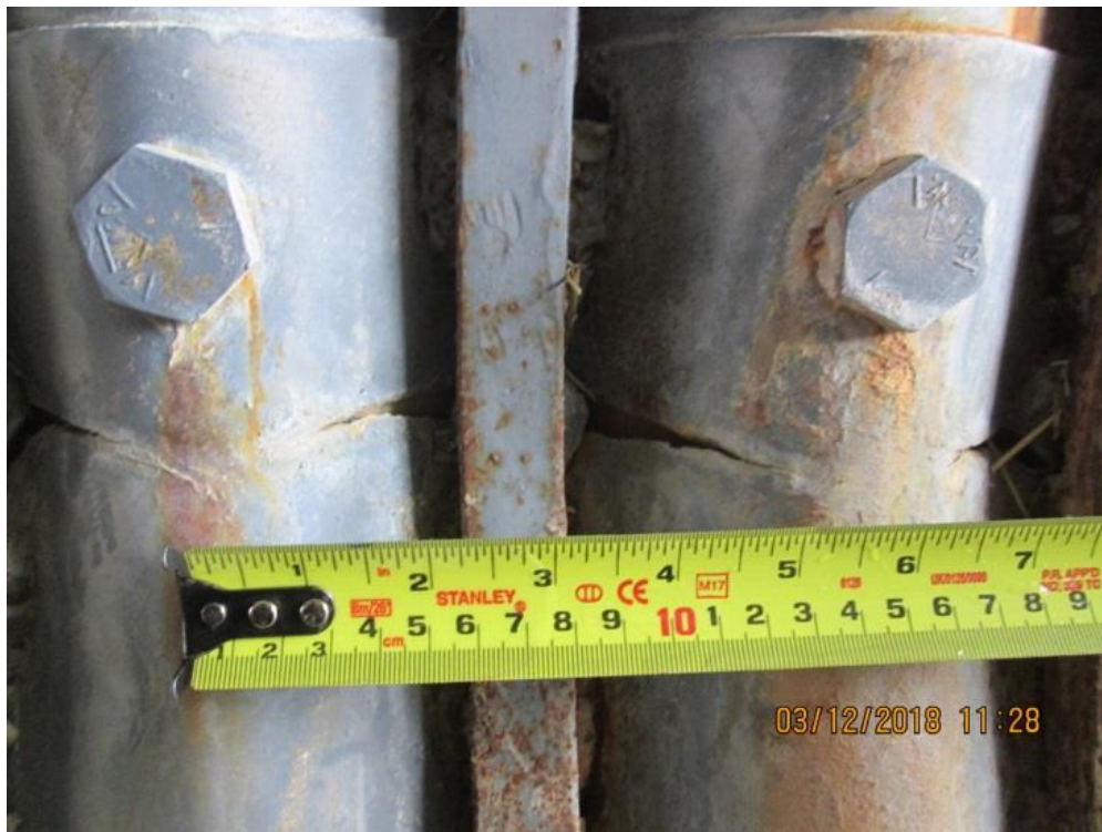
Cracking at springline along south side of structure
