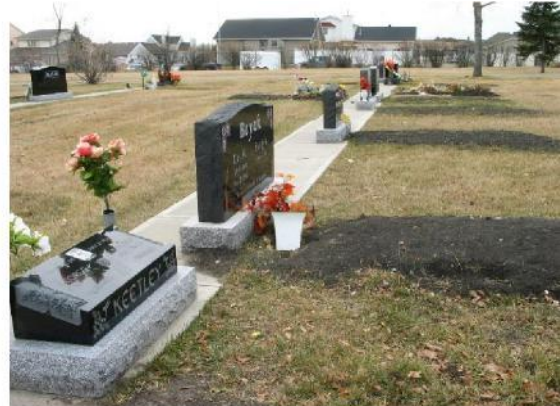
Concrete ribbon foundation for back-to-back casket lots without planting strip. (HLI design)
