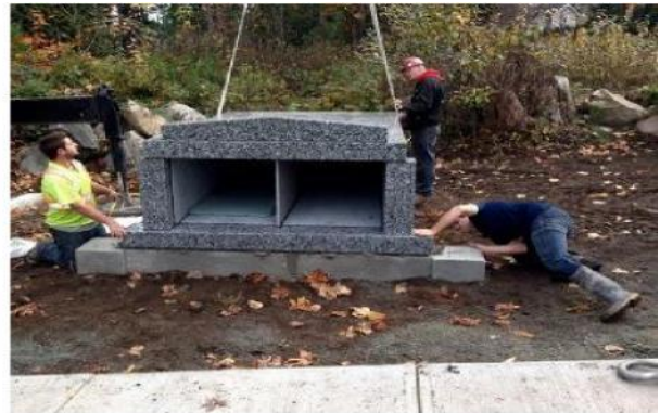
Installation of double lawn crypt
