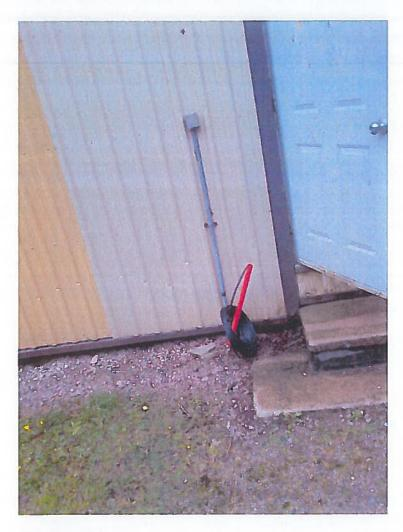
The cladding is in good condition. I would not recommend any addition or repair. There should be some cleanup around the building.
