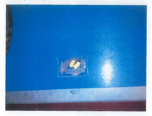
Two switches with no cover plates only duct tape.
