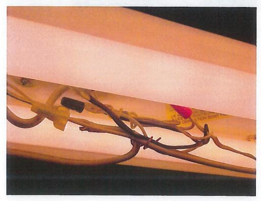
The next picture shows some of the lighting. The dome lights do not work. There is a broken bulb in the fixture on the left. One of the fluorescent lights at the side of the building did not work either.
