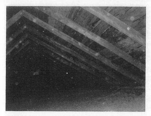
The roof structure over all appeared sound. There were some roof joists that were broken or had been repaired. There were cracks in some of the beams. The picture below shows one of the joists that has had a second board attached to it. There is evidence of water staining on the sheathing from the leaks in the roof as well. The beam that the joists are supported by looks sound. There is no obvious damage.
