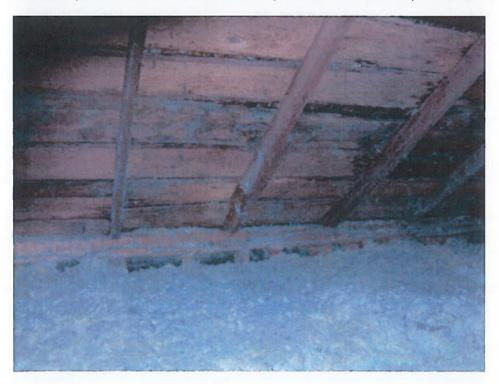
The next picture shows more of the structure. Two joists have had additional 2X6s spliced to them. The wall stud on the left does not reach to the beam.
