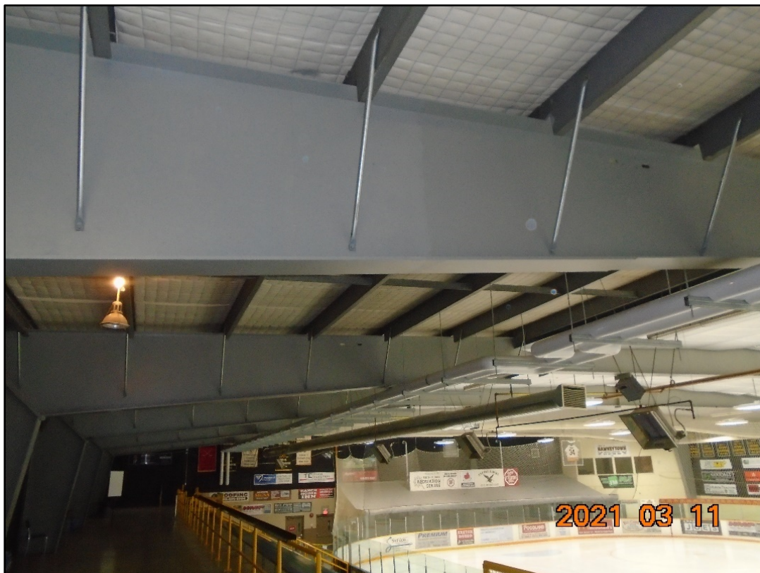
Typical Coating Condition
