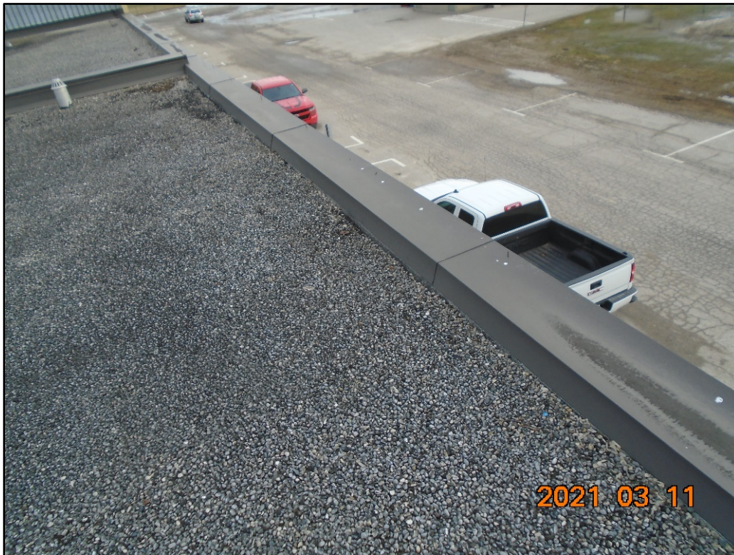
Loose Flashing Screws – East Wall of Hall
