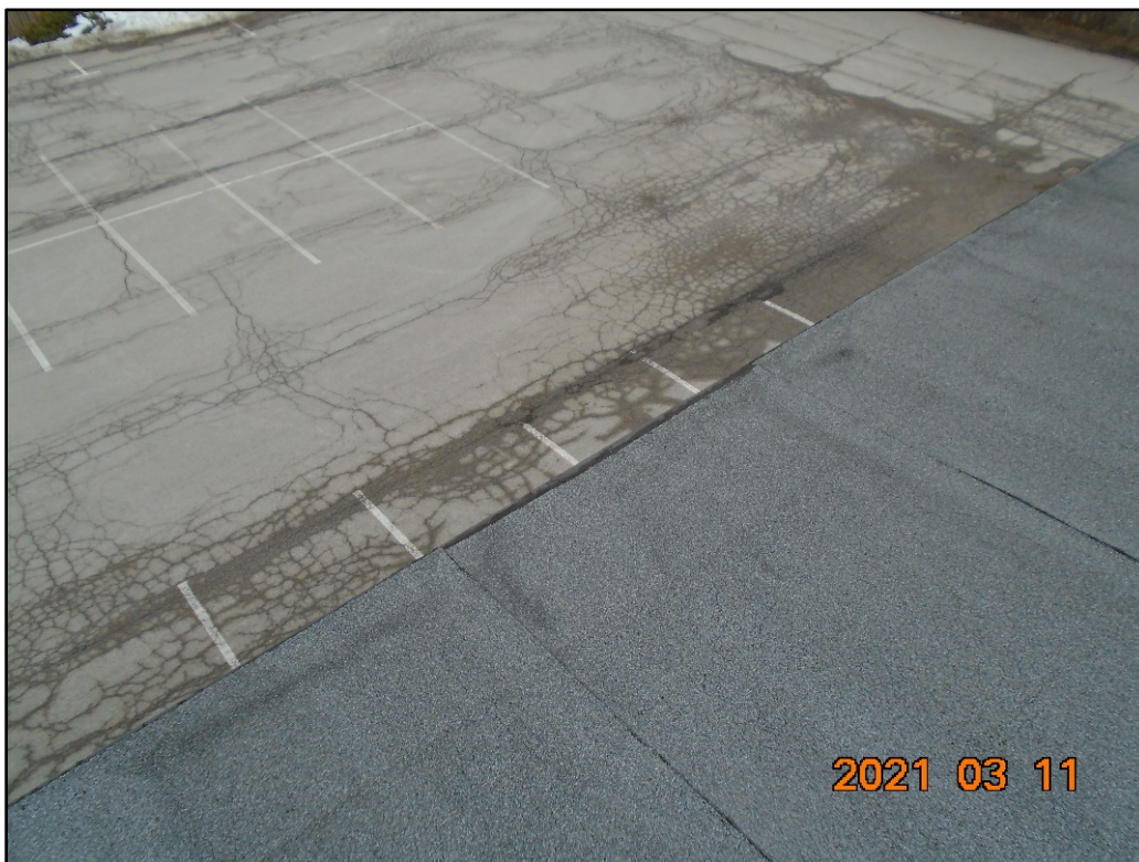
Gap Between Roofing and Flashing over Ice Surface – East Wall
