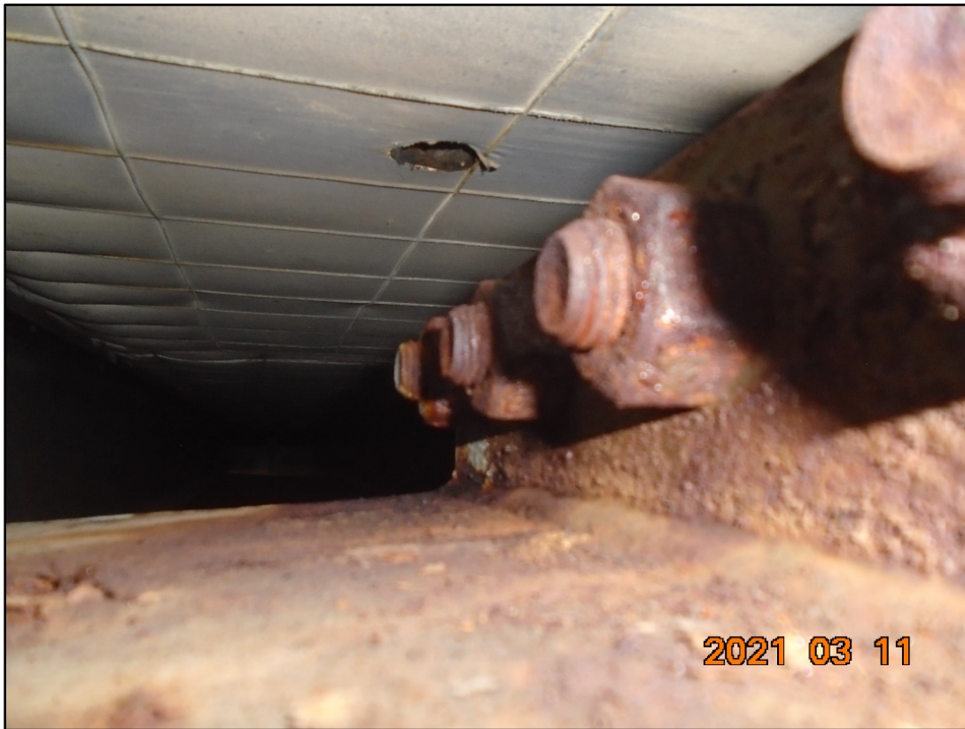
Bolts at Top of Beam Over Ice Surface
