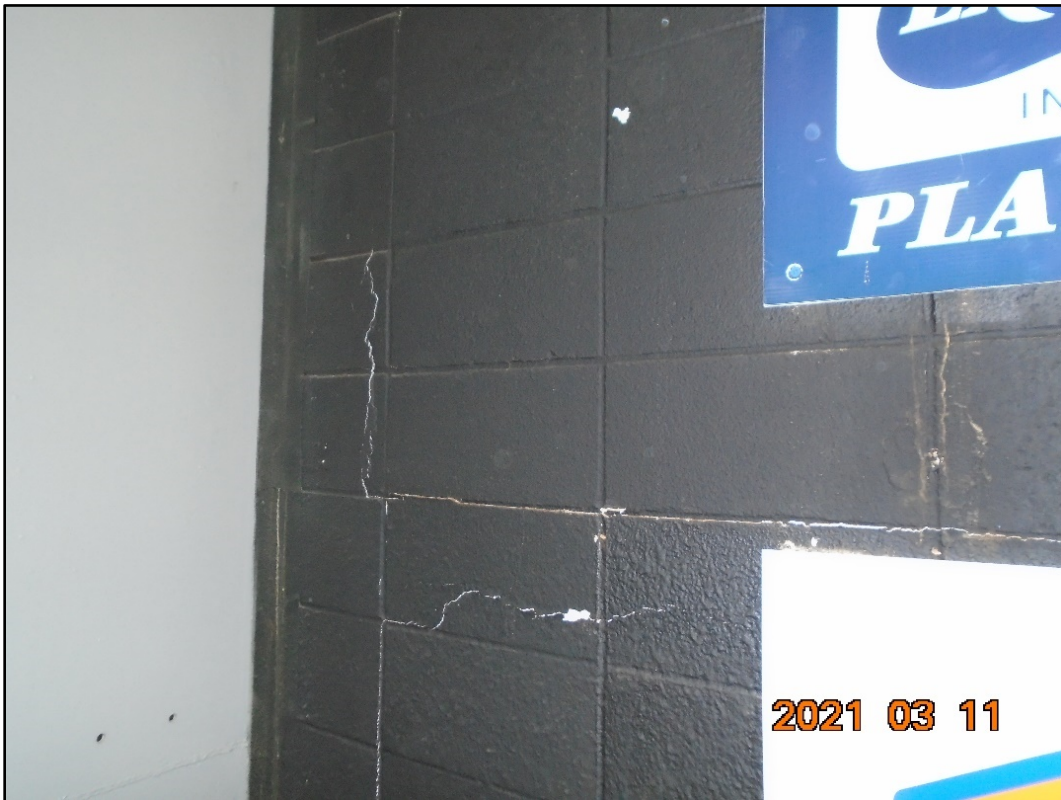
Cracking and Shear Ledge in West Masonry Wall of Ice Surface
