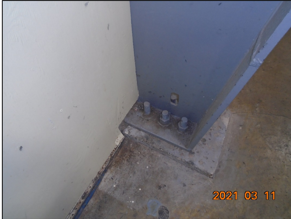
Missing Nut at Base of 7 th Column from North End Wall – West Side of Ice Surface
