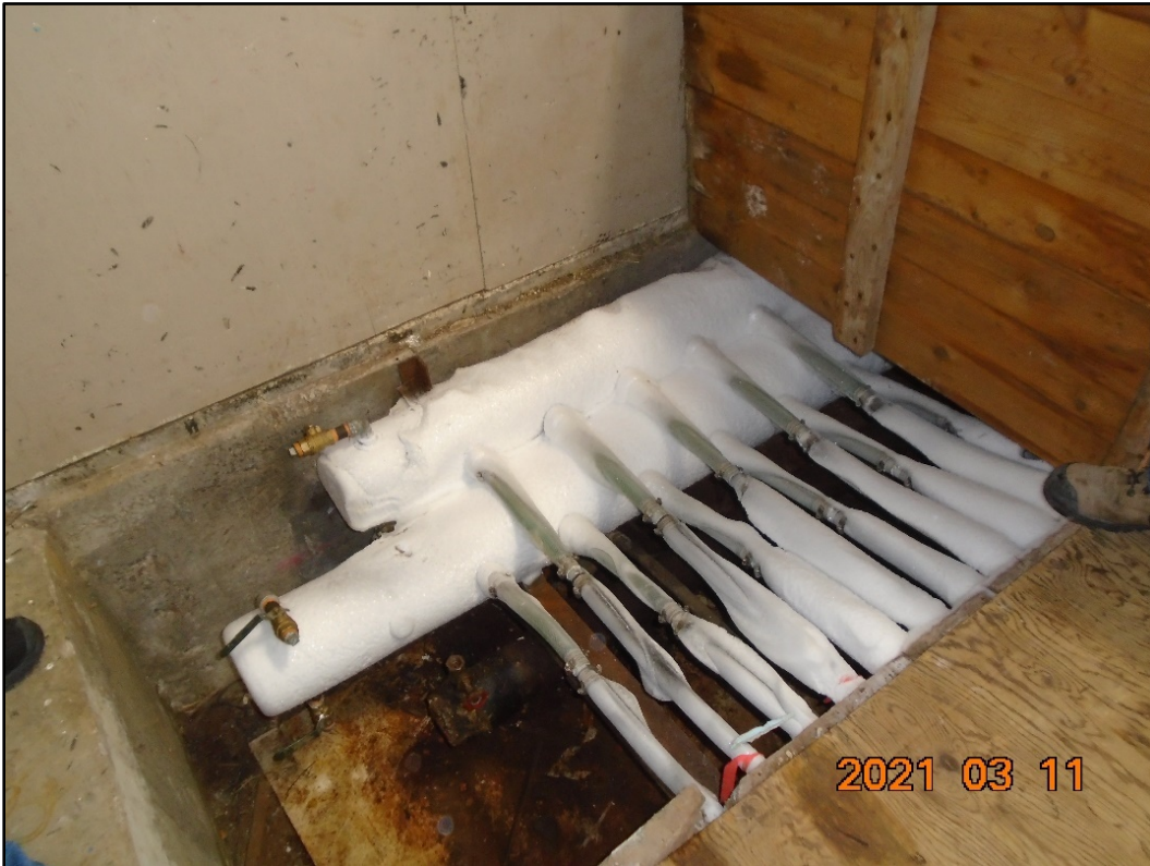
Header and Pipes for Ice Surface Cooling
