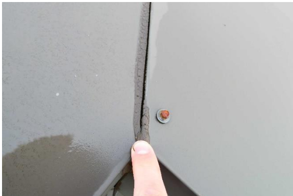
Photo Exhibit No. 32 Failed sealant joint at metal flashing, in location of standing water.
