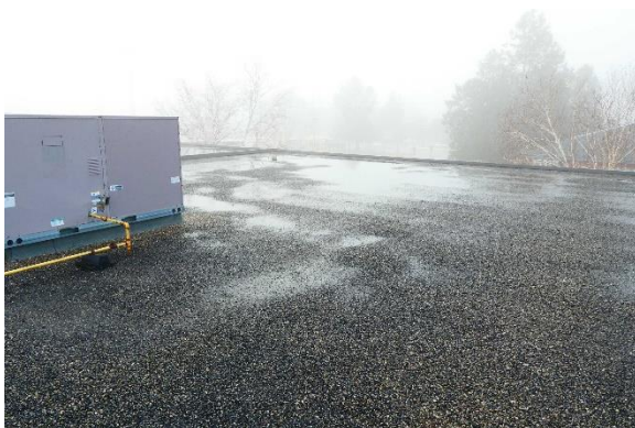
Photo Exhibit No. 27 Large area of ponding water.
