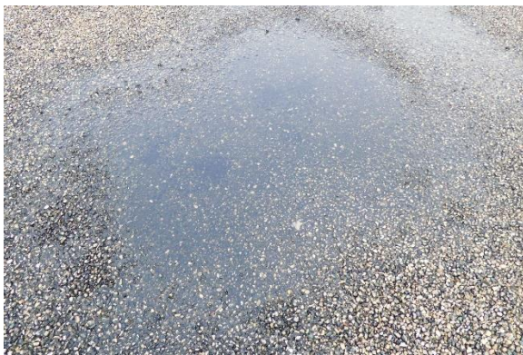
Photo Exhibit No. 26 Large area of ponding water.
