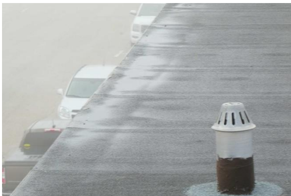
Photo Exhibit No. 15 Ponding water at roof edge.
