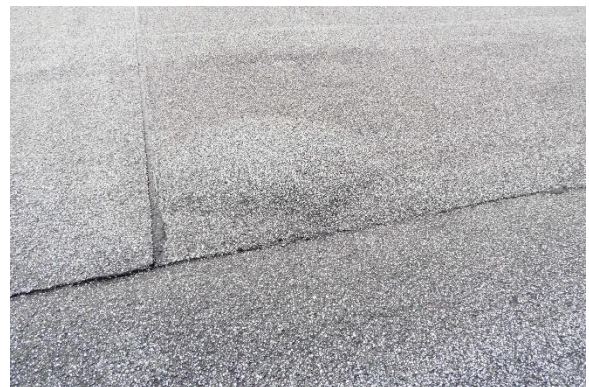
Photo Exhibit No. 12 Large blister beneath cap sheet.
