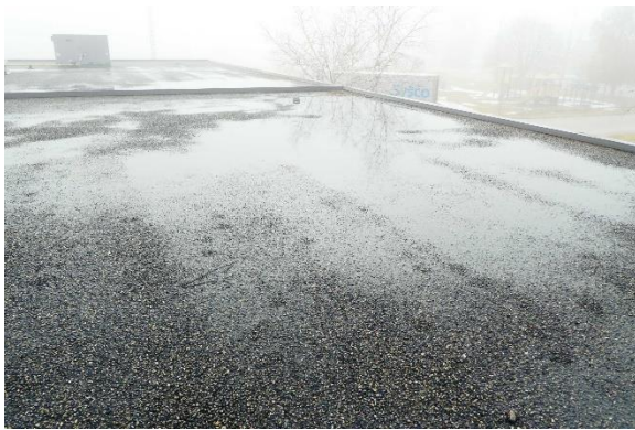
Photo Exhibit No. 25 Large area of ponding water.
