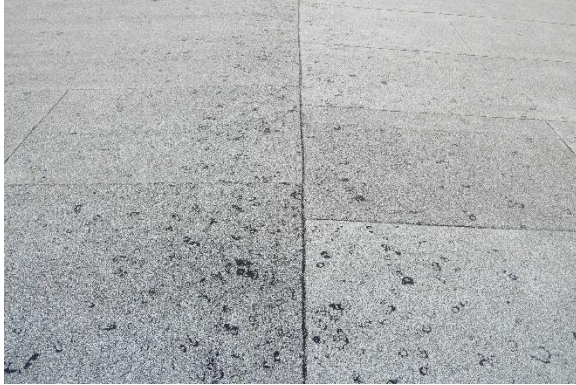
Photo Exhibit No. 7 Large hail strikes on the roof.
