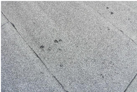
Photo Exhibit No. 8 Large hail strikes on the roof.
