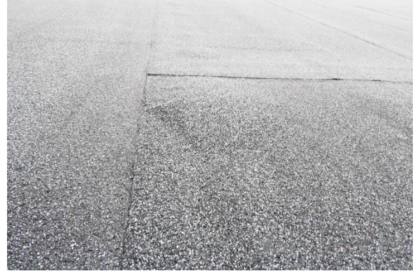
Photo Exhibit No. 10 Large blister beneath cap sheet.
