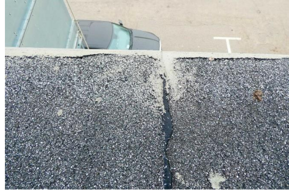
Photo Exhibit No. 16 Failure of sealant/repair.
