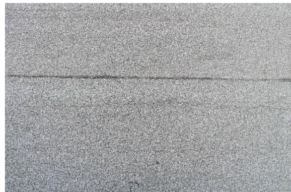
Photo Exhibit No. 18 Alligatoring/damaged cap sheet membrane.
