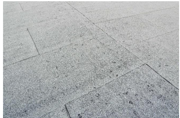
Photo Exhibit No. 5 Large amount of hail damage present on roof.
