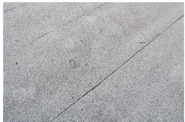
Photo Exhibit No. 6 Large hail strikes on the roof.
