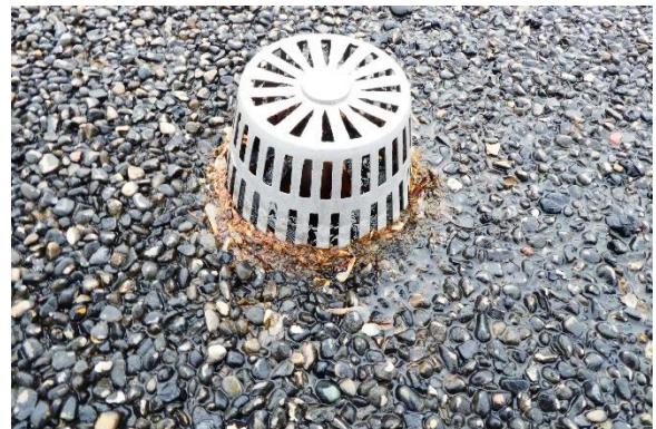
Photo Exhibit No. 36 Growth/debris at drain preventing drainage of water.
