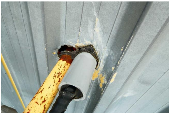
Photo Exhibit No. 33 Large gap in the metal at pipe penetration above recreation center roof.
