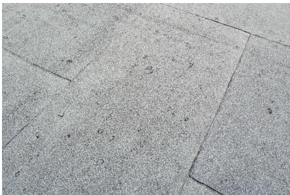
Photo Exhibit No. 9 Large hail strikes on the roof.
