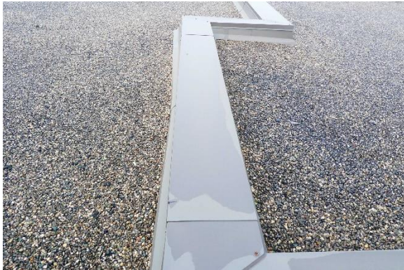
Photo Exhibit No. 31 Nearly flat metal flashing, note standing water.
