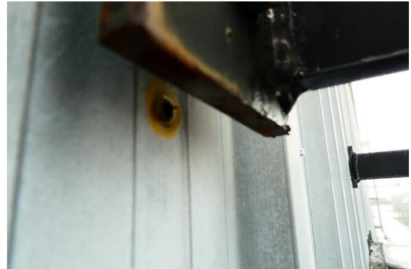
Photo Exhibit No. 34 Fastener hole in metal above recreation center roof.
