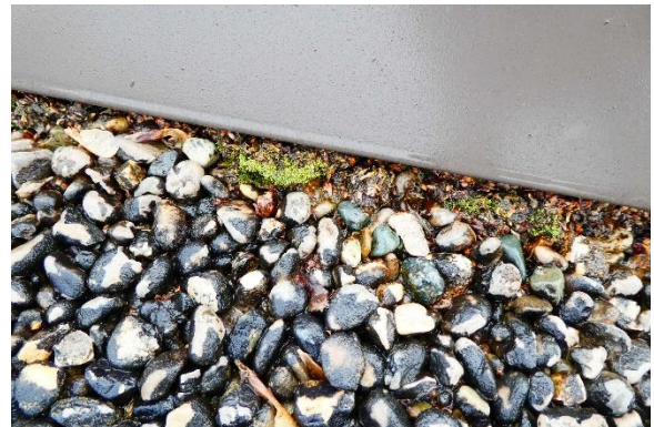
Photo Exhibit No. 35 Organic growth at/beneath metal flashing.
