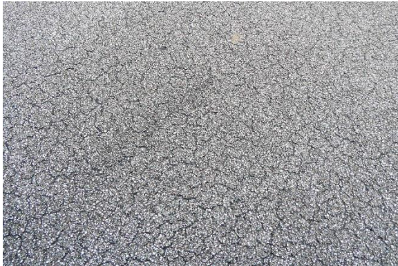
Photo Exhibit No. 20 Alligatoring/damaged cap sheet membrane.
