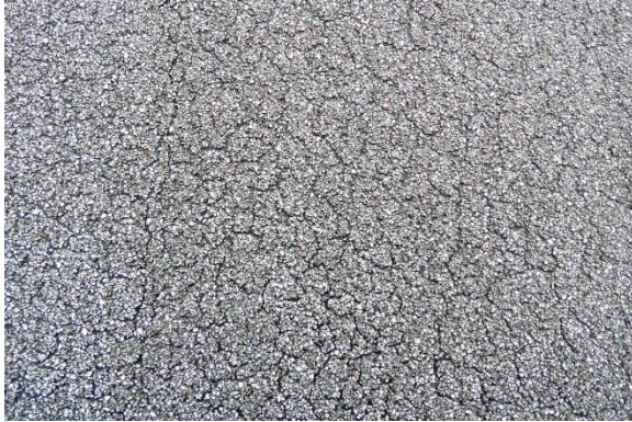
Photo Exhibit No. 19 Alligatoring/damaged cap sheet membrane.
