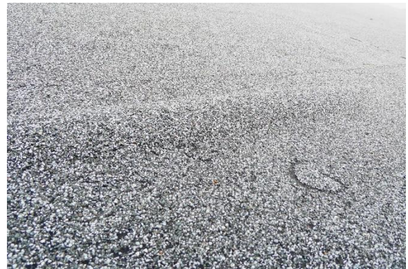
Photo Exhibit No. 11 Large blister beneath cap sheet.
