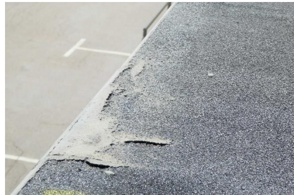
Photo Exhibit No. 17 Failure of sealant/repair.
