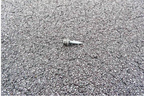
Photo Exhibit No. 13 Fastener/debris on roof area.
