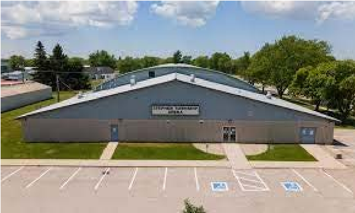
Source: Municipality of South Huron
