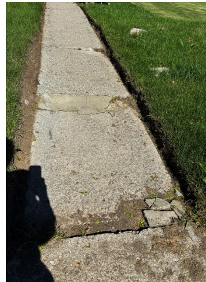
Current condition of walkway from street
